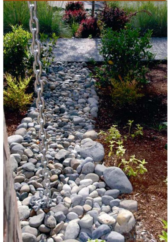
This shallow **conveyance trench** is letting water soak into the soil, while it carries excess from big storms to a pipe running under the sidewalk, to a street drain.
