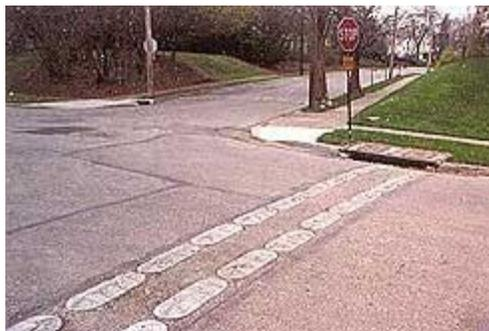
**Rumble Strips** – Rumble Strips, along with speed humps, raised crosswalks and speed tables, are designed to slow traffic to negotiate the device. Rumble Strips are normally placed at crosswalks.
